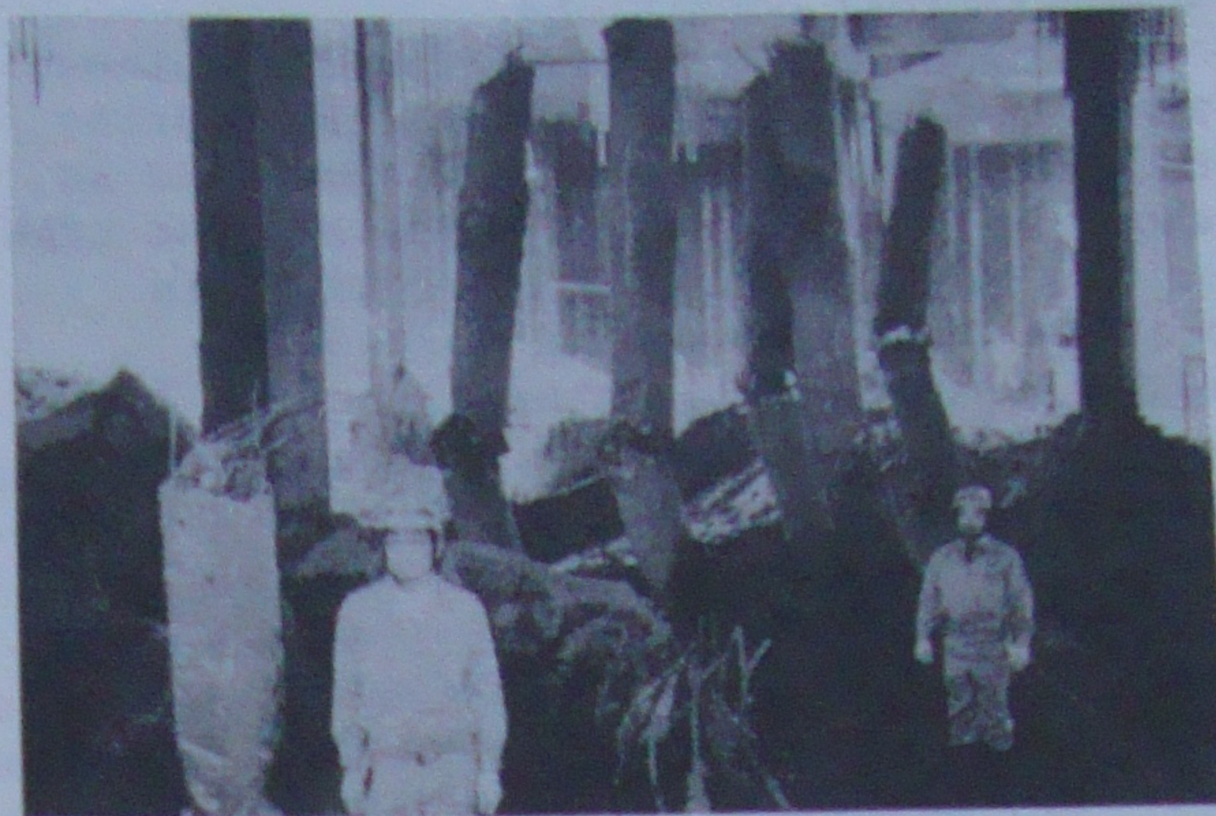
Photo 4 Damage to RC pile
